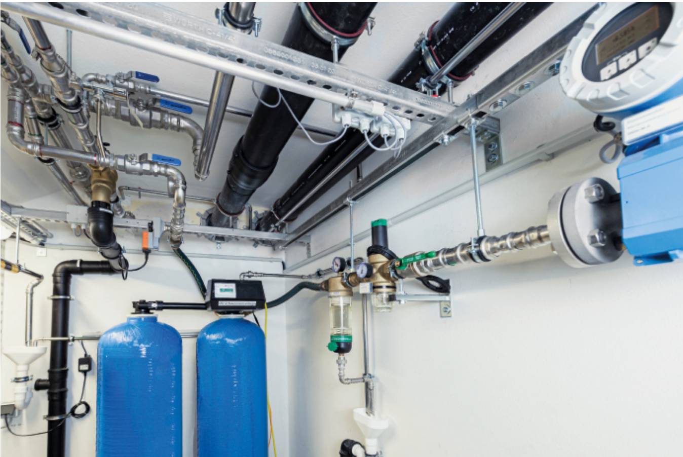
› Double water softening unit to remove the minerals that form lime scale and dosing station for inhibitors to prevent corrosion, integrated into a container unit
